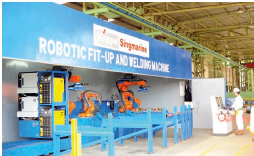
The robotic welding machine at Keppel Singmarine uses 25% less man-hours compared to the manual fabrication of pipe spools
